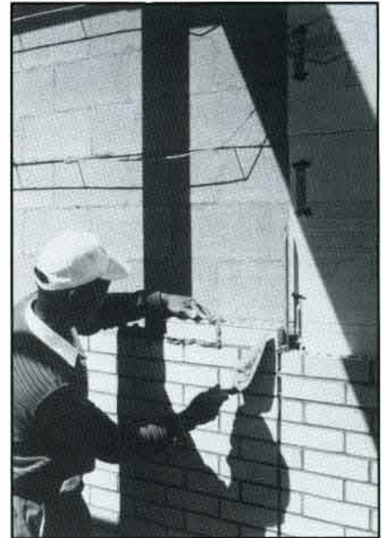
The brick veneer goes up right over the STYROFOAM brand insulation. STYROFOAM brand insulation is highly water resistant and exposure to the elements on the job site will not cause damage.
