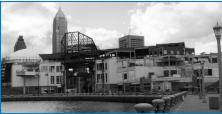
Approximately 18,000 square feet of STYROFOAM brand Square Edge insulation were used to insulate the stone-faced walls of the museum.
