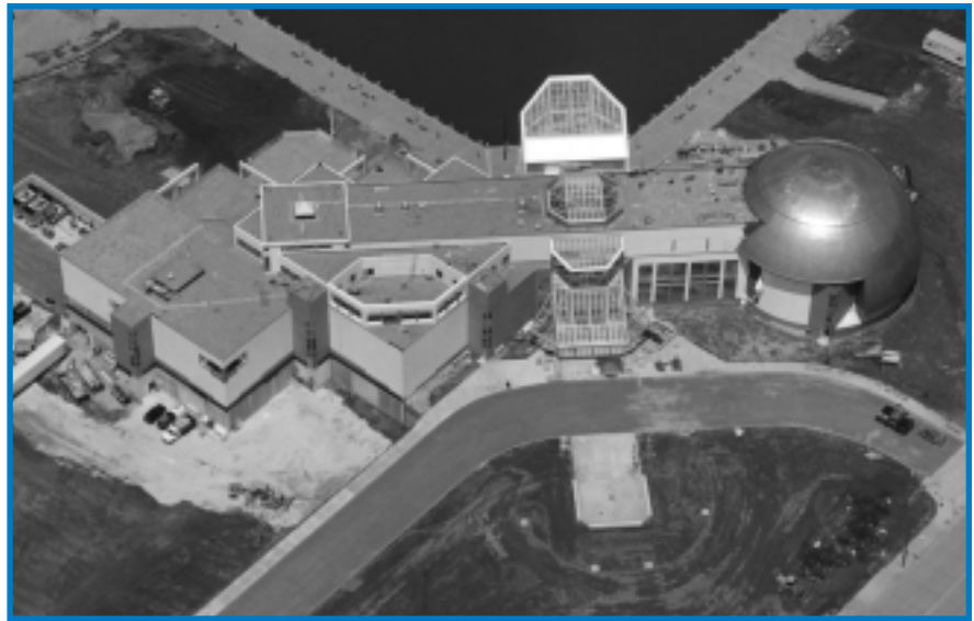
A single-ply, ballasted system using tapered thicknesses of STYROFOAM brand insulation covers the concrete and metal deck roofs of the museum.
